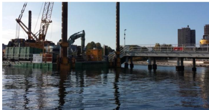
Fig. 8: Harbour construction-site in Kiel-Schilksee
